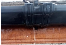
Figure 2 a: Leaking Gutter
